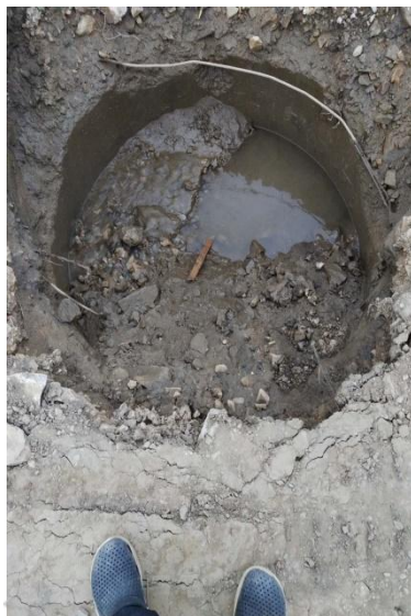
Sewer Chamber Blocked
