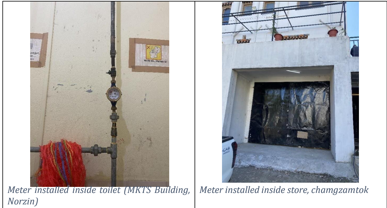
Figure no 6: improper location of meter
