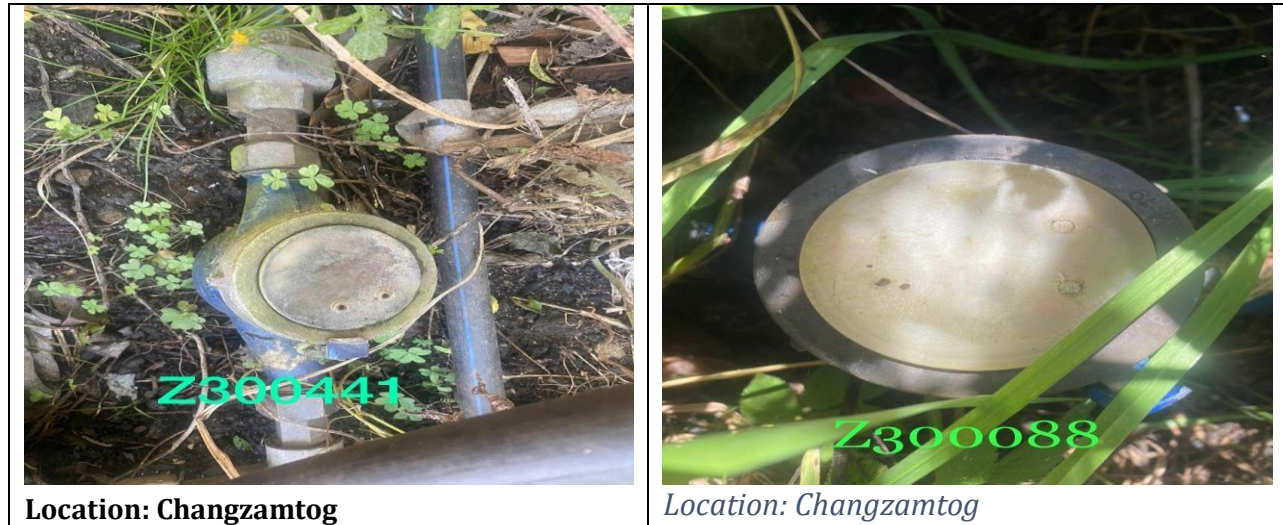
Figure No 5: Unclear water reading display
