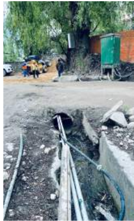
Small humepipe drains like this one blocks easily because it is used to lay private water pipes.
