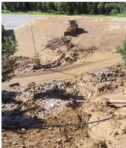
Landslide washing away water lines
