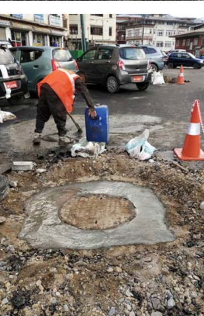
Raising and lowering of manholes in various locations
