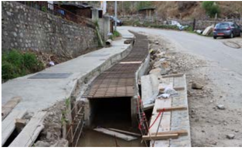
Drain reconstruction in Gida Lam
