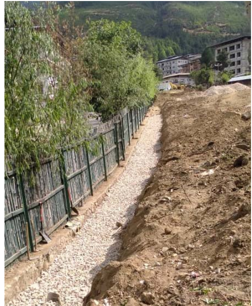
French drain construction
