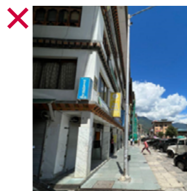
Obstructions within footpath
