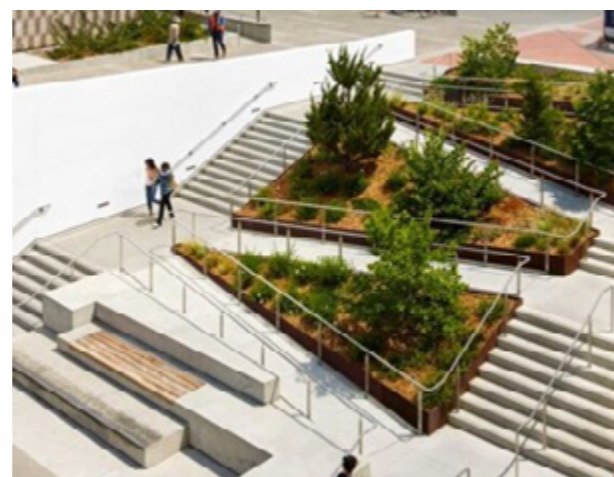
Inclusion of accessible ramps Source: Clay Holden
