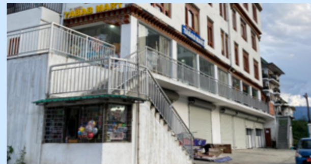
Significant level changes
