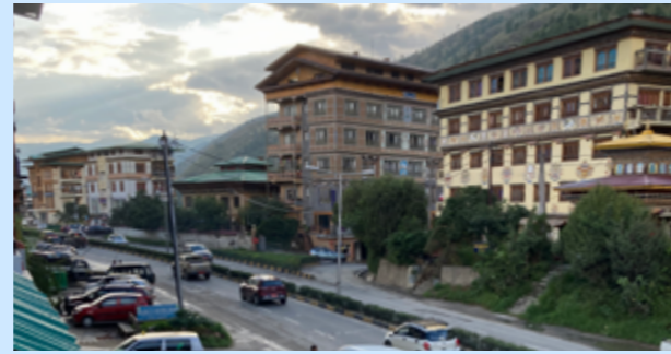
Express way forms a barrier to pedestrian movement
