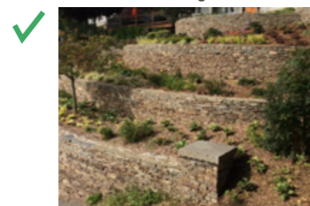
Stepped retaining wall faced with masonry and with planting areas interspersed
