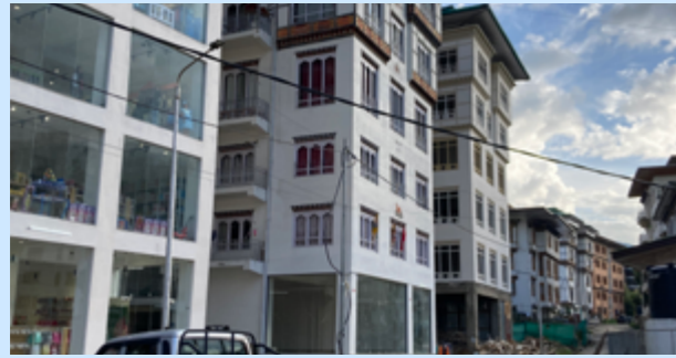
Congested developments and intensive commercial uses
