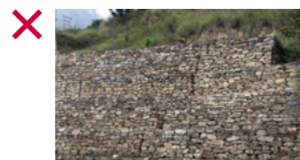
Monolithic retaining wall
